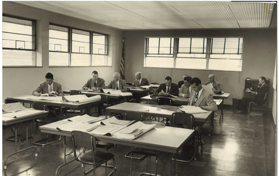
The magazine reported that the new plan room “is perhaps the most important room in the building. Quite a jump from that dingy room at the old quarters! ... and look at that ceiling. The entire ceiling is a honeycomb of baffles diffusing the light of seven rows of fluorescent tubes. That Modernfold door at the east end can be pushed back to open the entire end of the room facing the lounge when there is call for such an occasion.”
